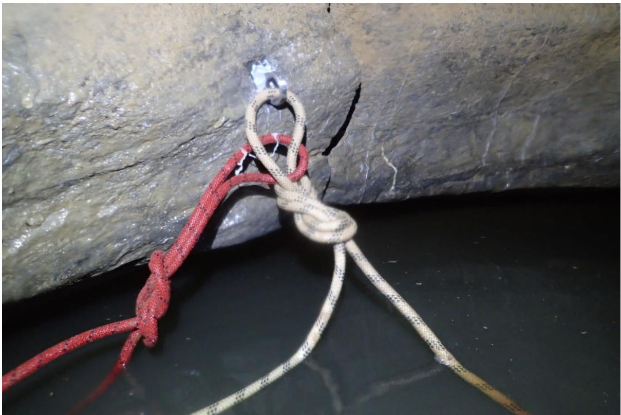
4. New anchor with white dive line to Sump 3 and red back-up line to natural belay and Sump 2 (St John's Bell)
