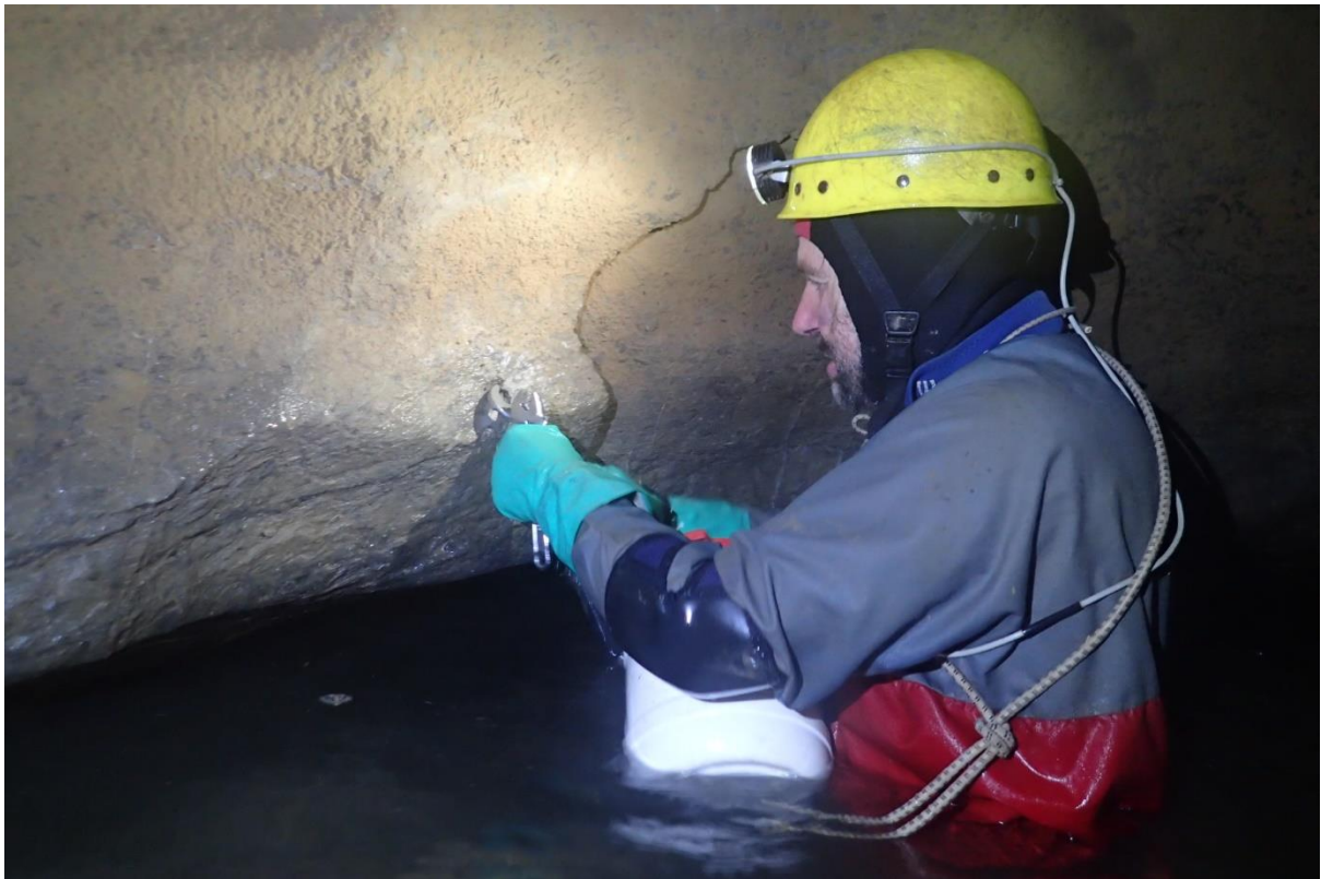
1. Removing old anchor
