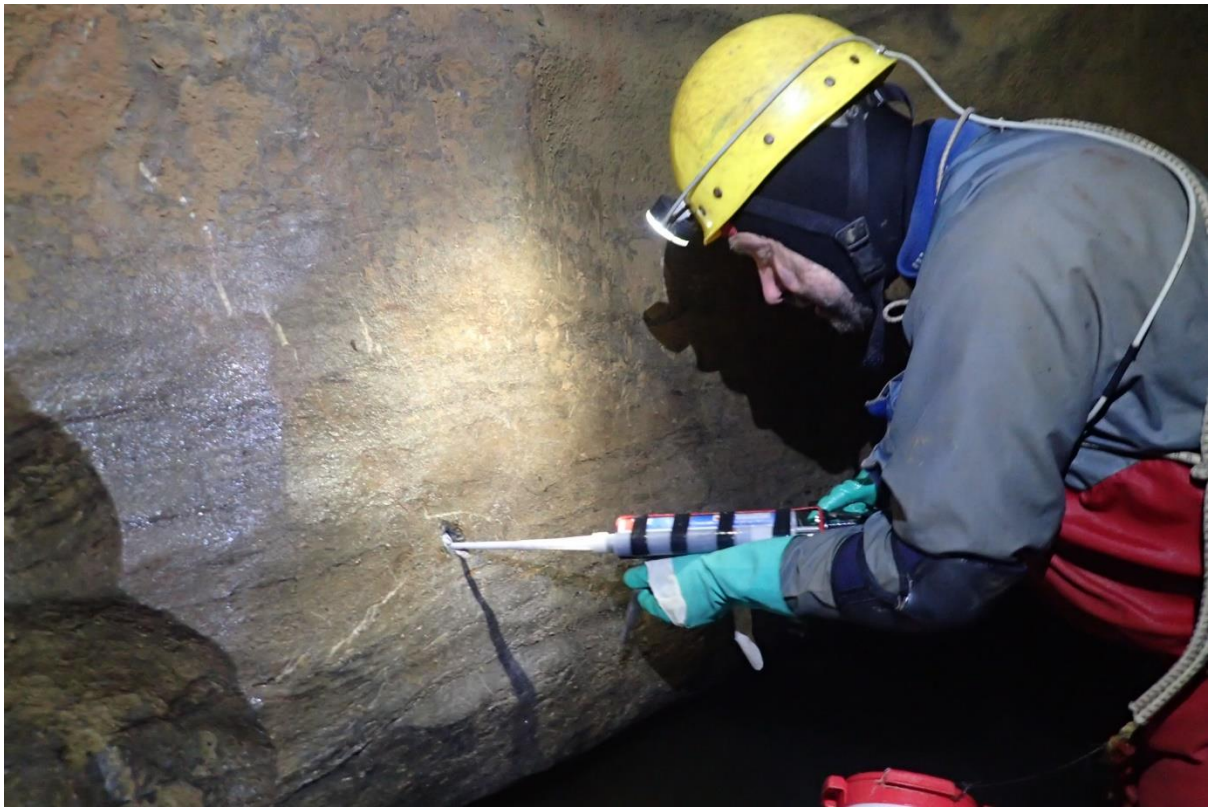
3. Placing resin for new anchor (Great Bell)
