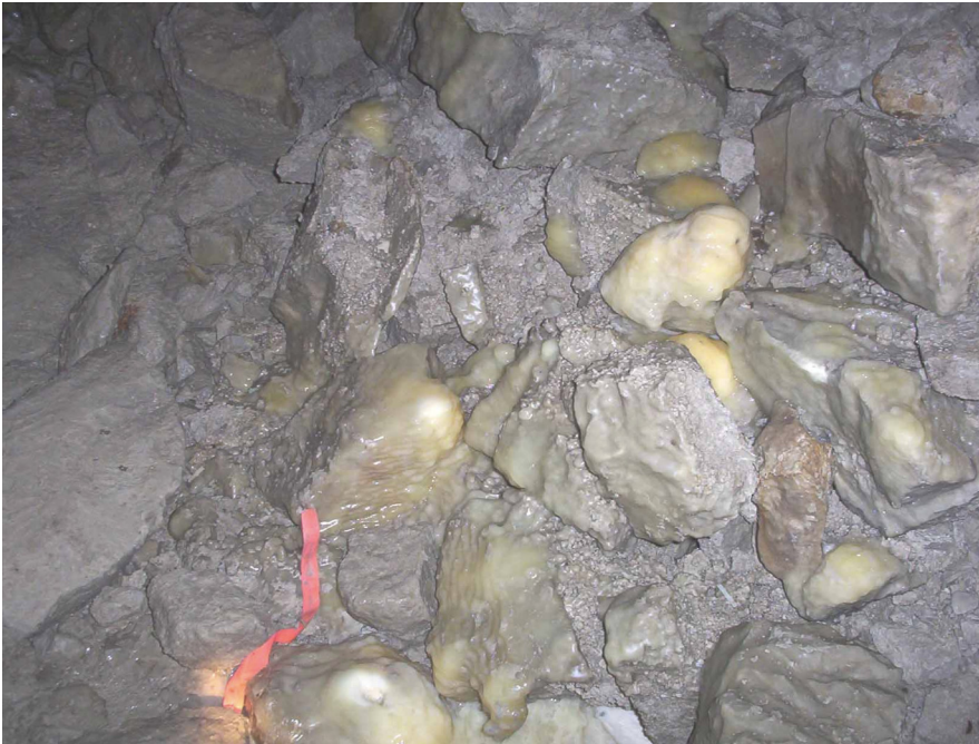
Some calcite deposits in excellent condition but inadequately taped.
