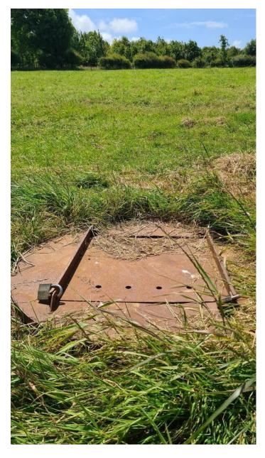
A report was received from the MCG that the lid for Cow Hole (Ubley Hill area) was in a poor state. An inspection was conducted and the lid does have some issues. The hinges are pretty much seized, the lid frame is not secured and thus the whole lid and frame can be lifted, the lid is bowed and the top concrete tube has started to crumble away. Most of this is probably due to it being run over by a tractor.
